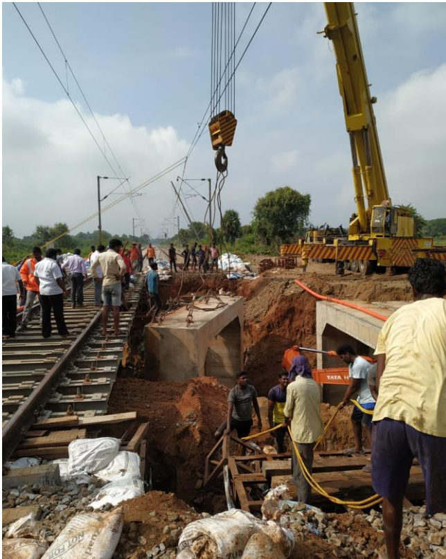
Preparation & Box Placing by Contractor
