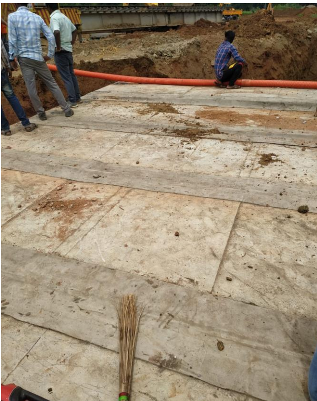
Patched installed in day shift
