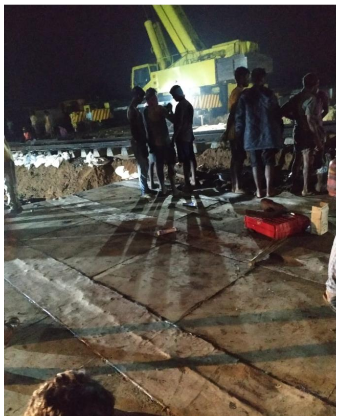
Patched installed in night shift
