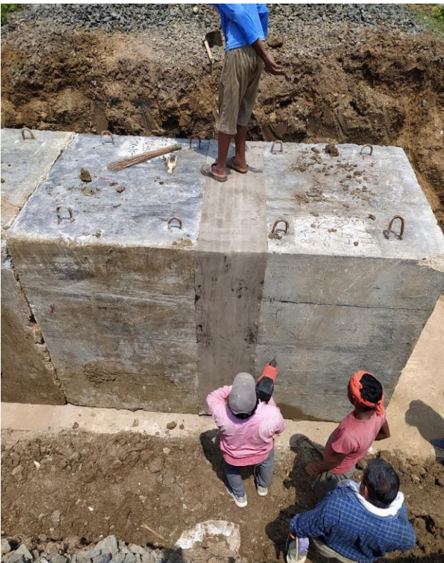
CC installation with Hilti Gun Nailing
