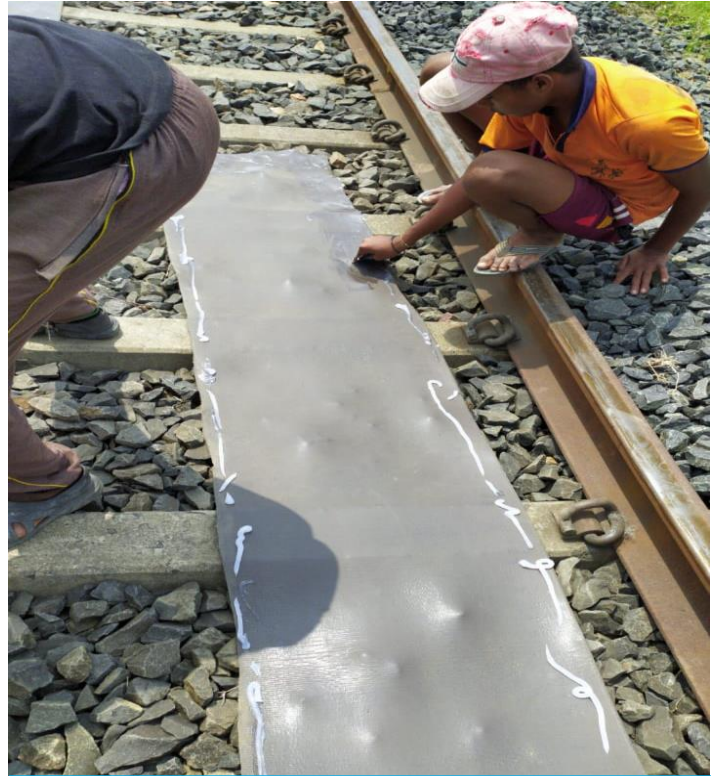
Cement Bases Silicon Sealant for Sticking of boxes
