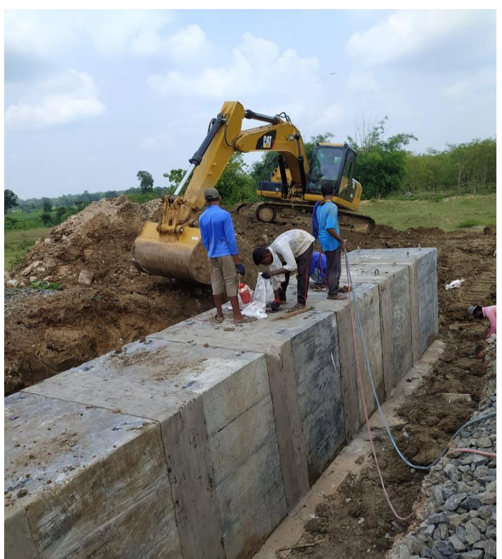
Complete Installation Photos
