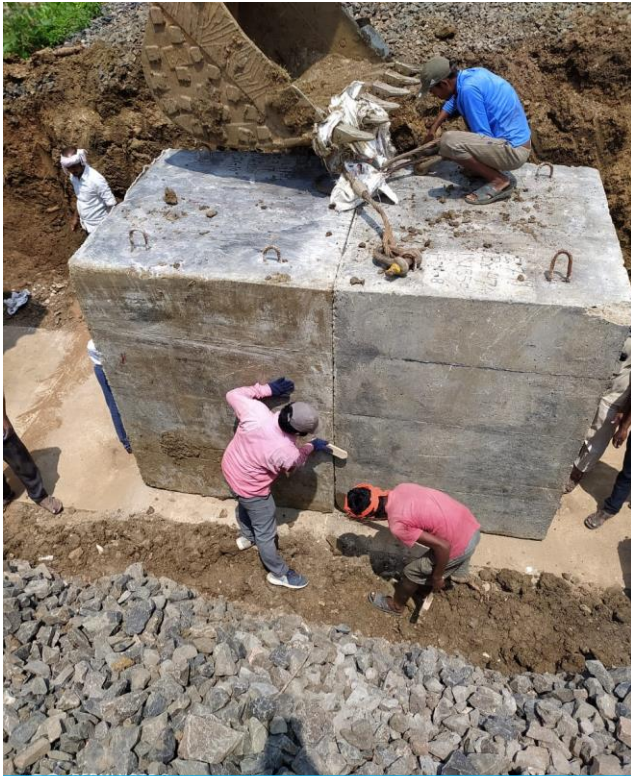
Cleaning Concrete Boxes before CC
