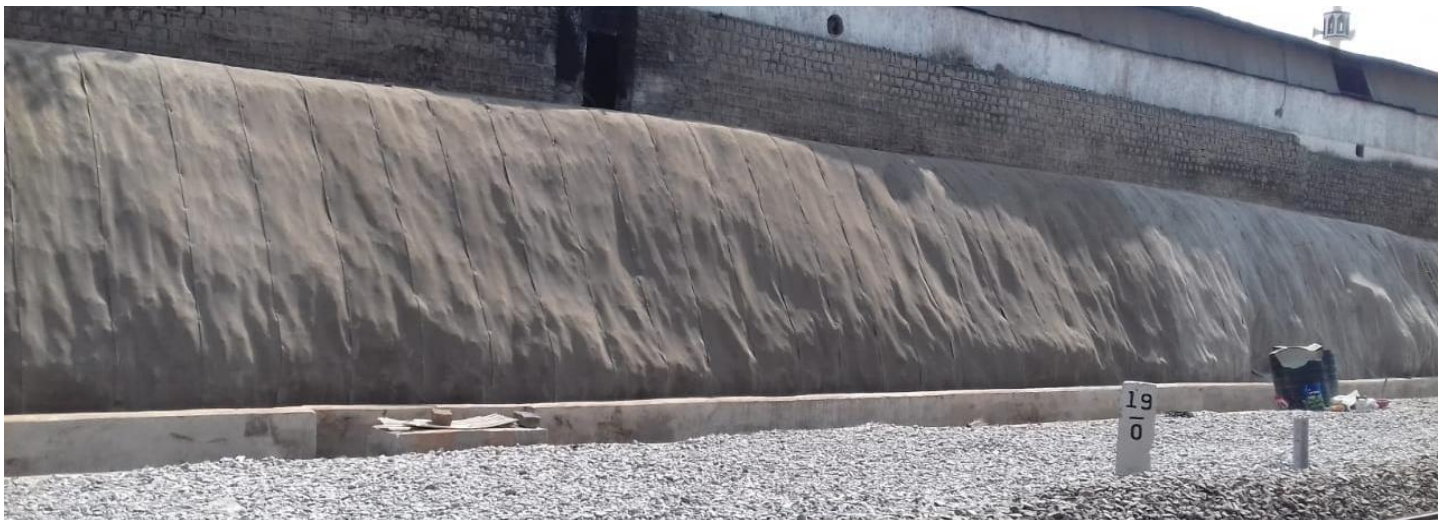
Site after Installation
