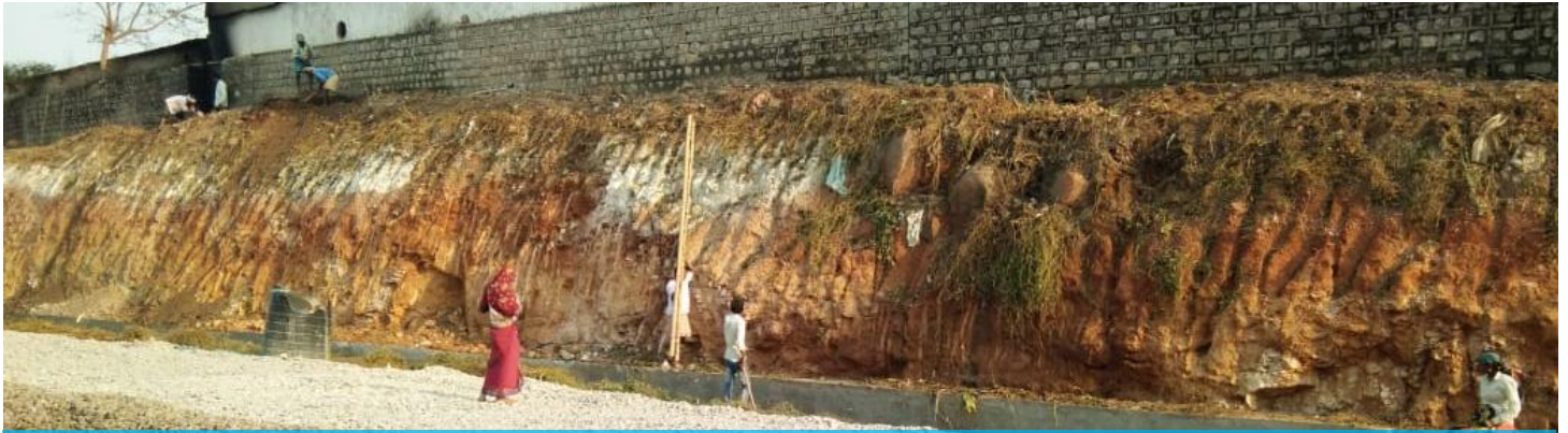
Site Before Preparation
