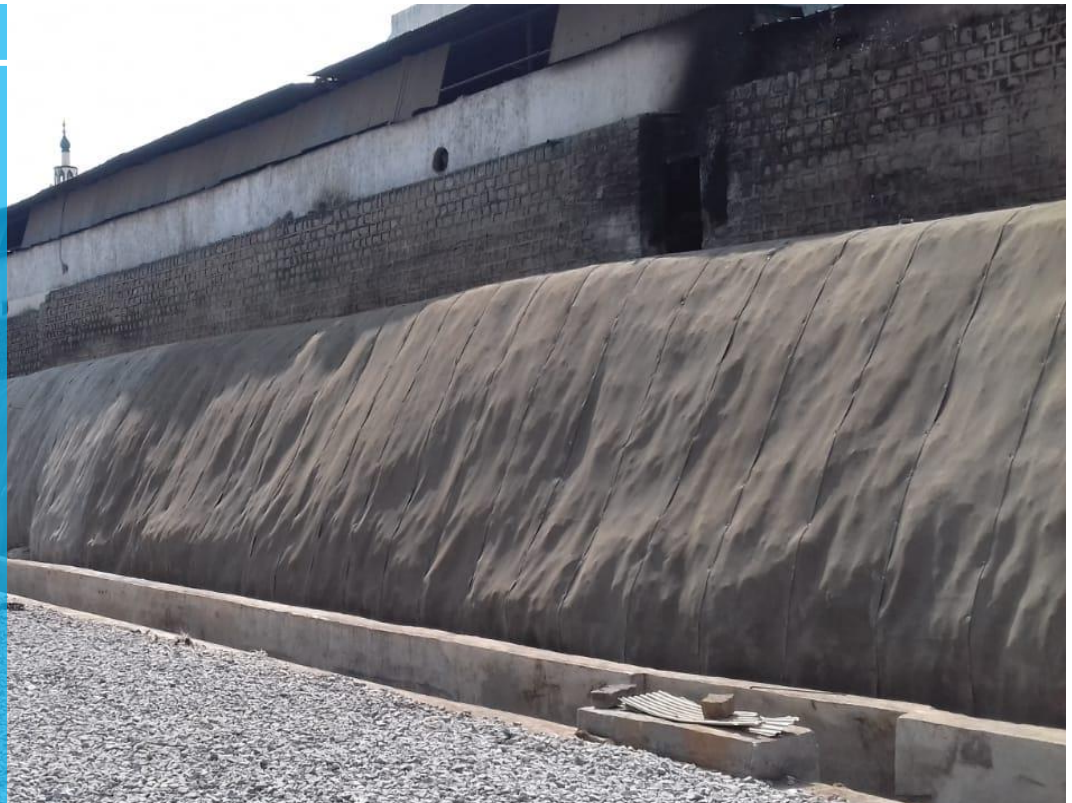
Installation Completion Photo
