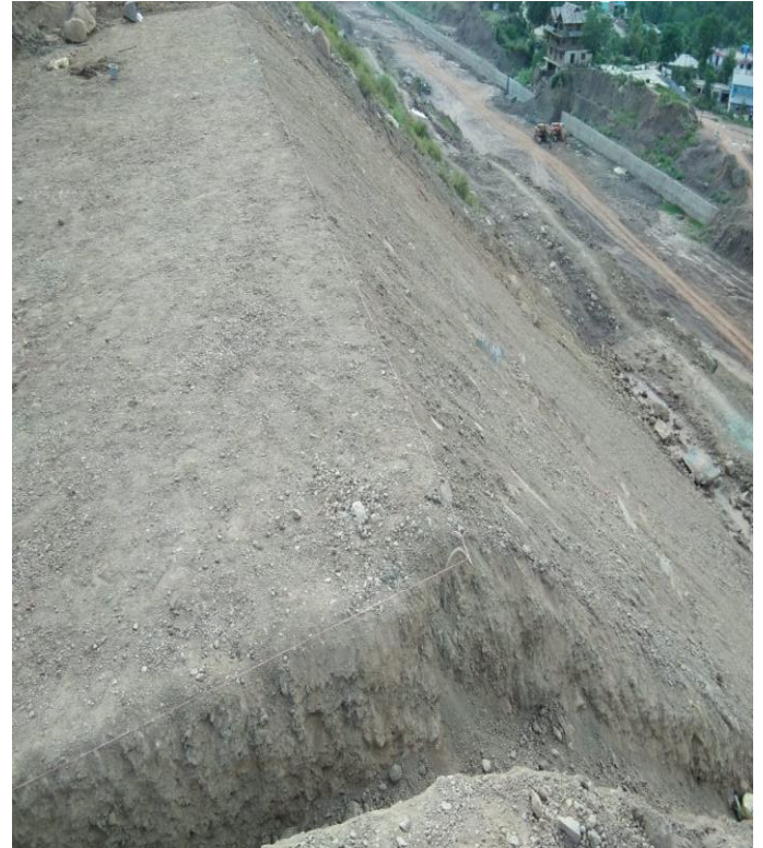
After Site Preparation
