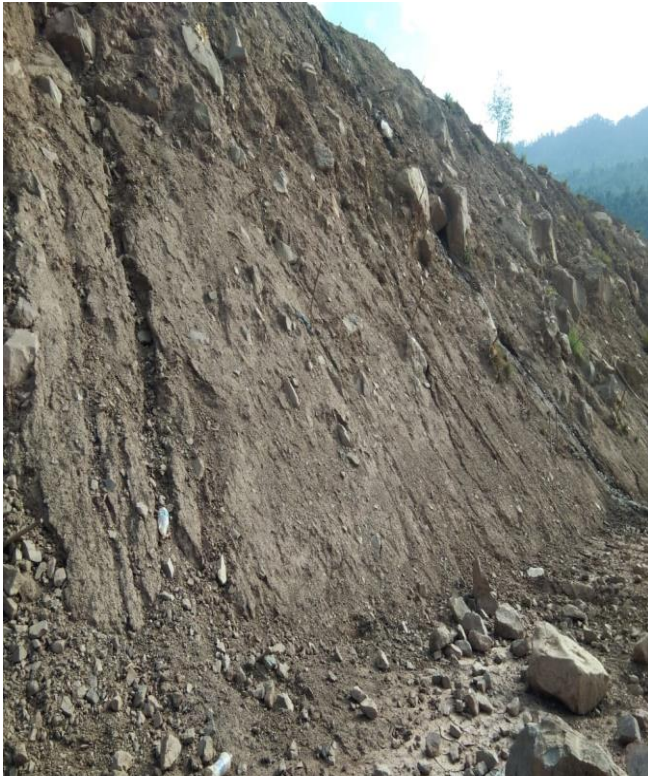
Before Site Preparation
