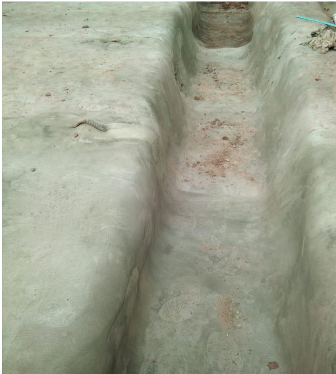
Catch Water Drain on Berm
