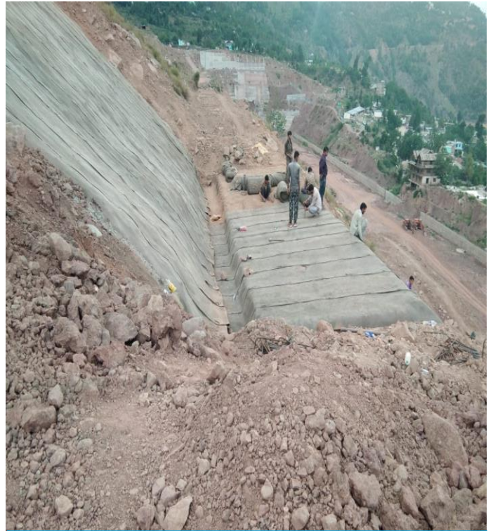
Middle Berm View
