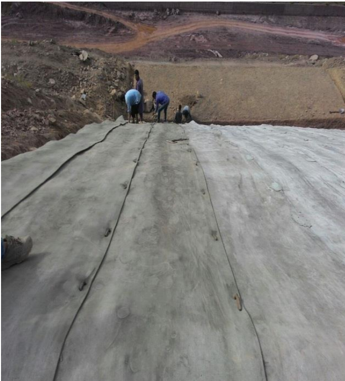
Laying of CC8
