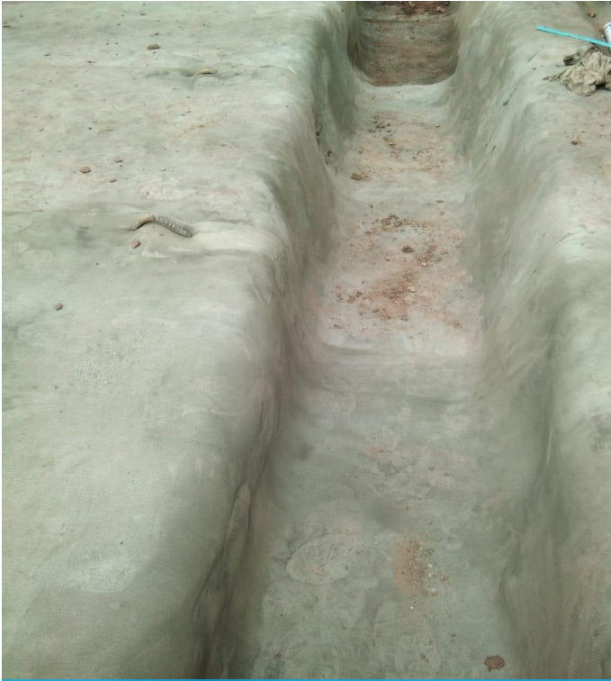
Catch Water Drain on Berm
