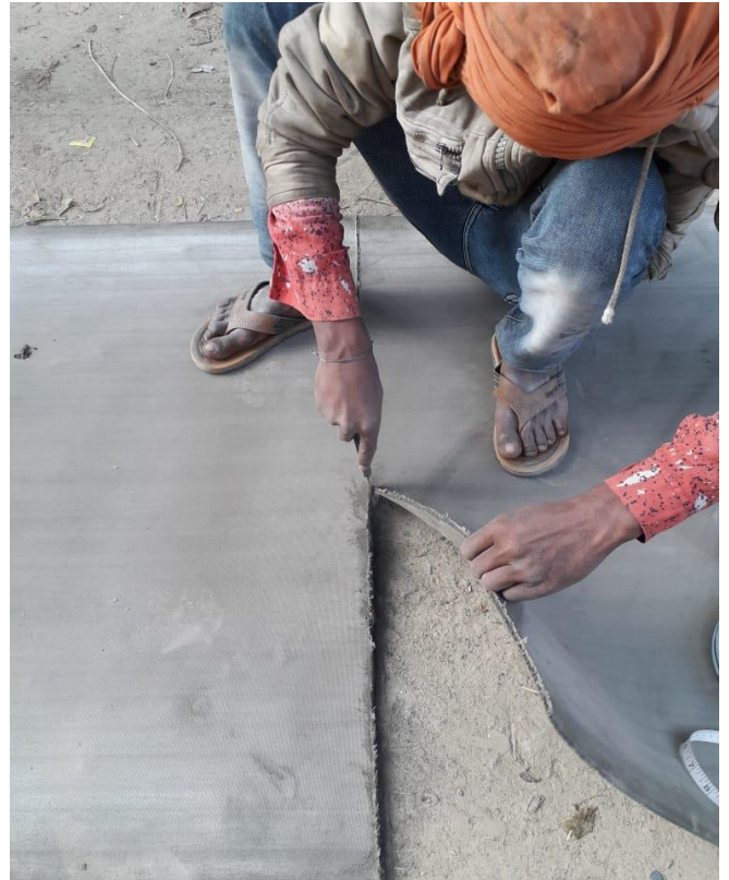
Cutting of CC patch in required dimensions
