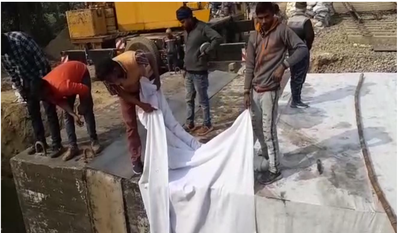
Covering CC Patches & Joints with Geomat / HDPE sheet
