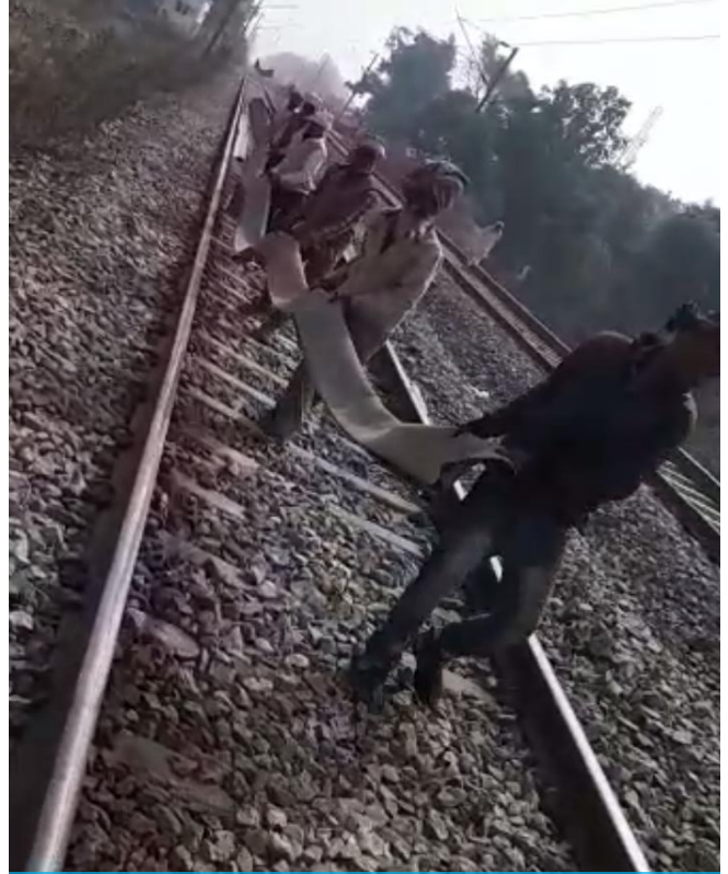
Cutting of CC patch in required dimensions
