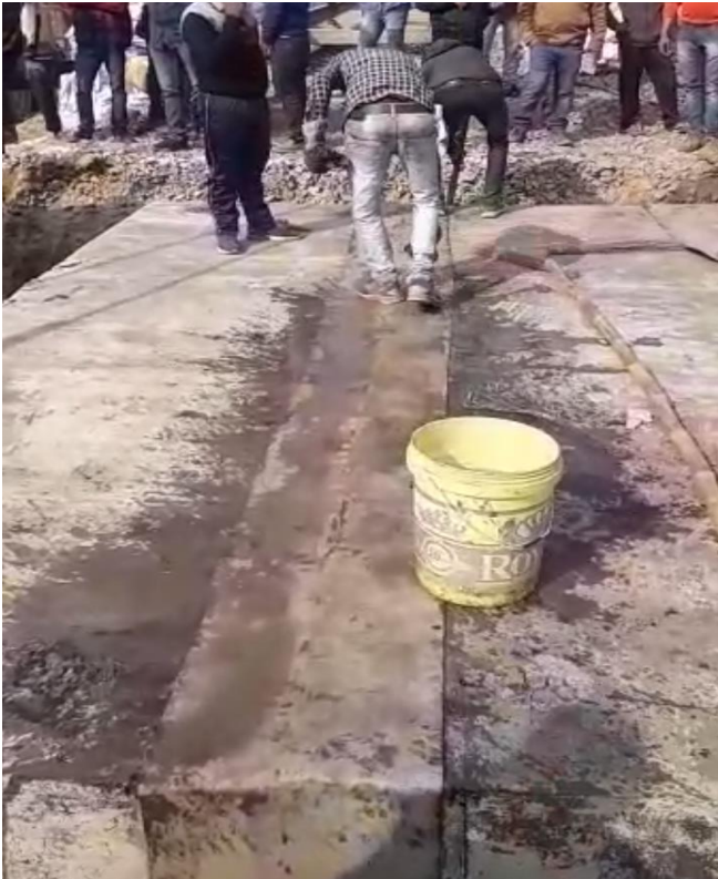
Cleaning of Dust from Joints
