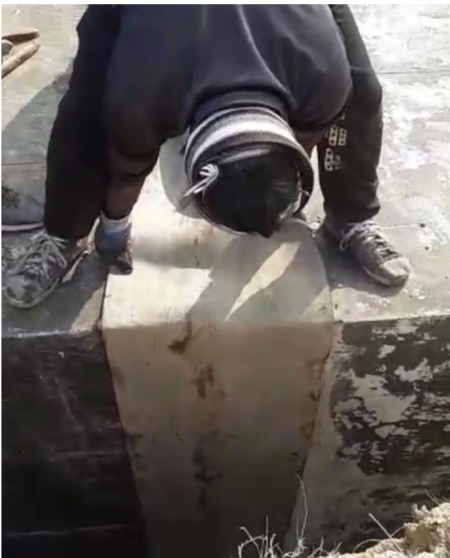
Placement of CC patch over Joint
