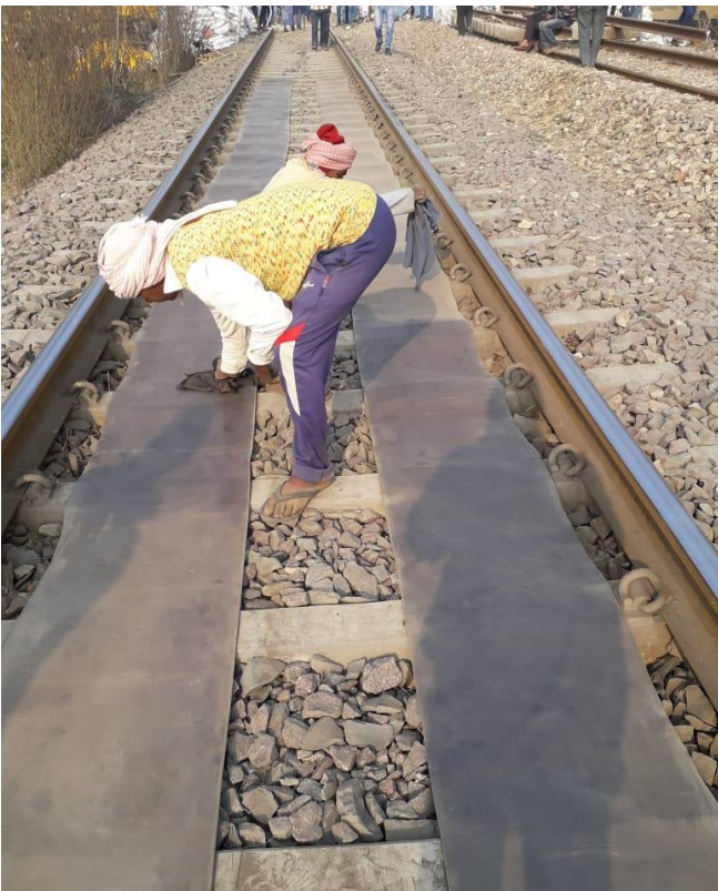
Cleaning of PVC portion
