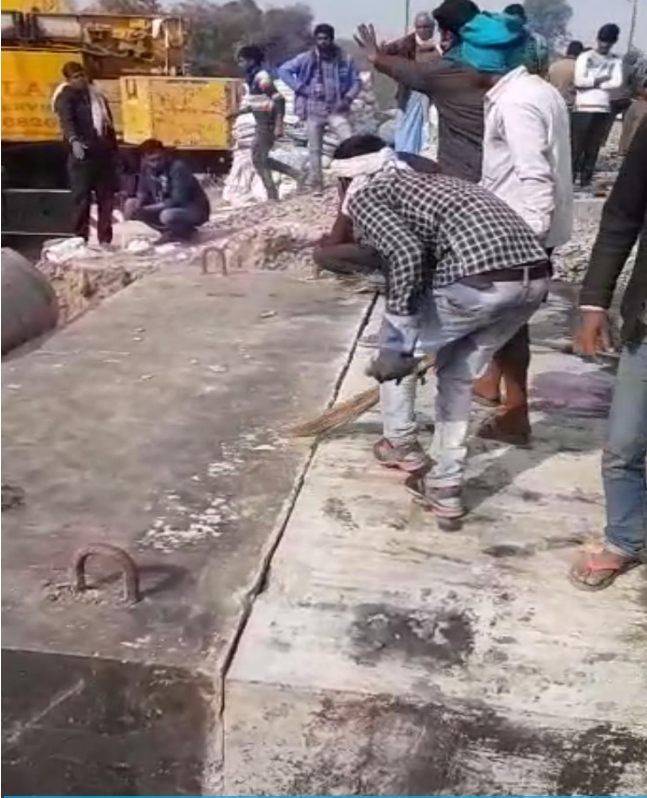
Cleaning of Dust from Joints
