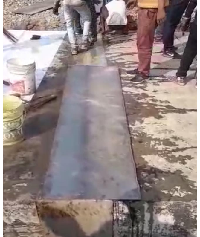
Cutting of CC patch in required dimensions
