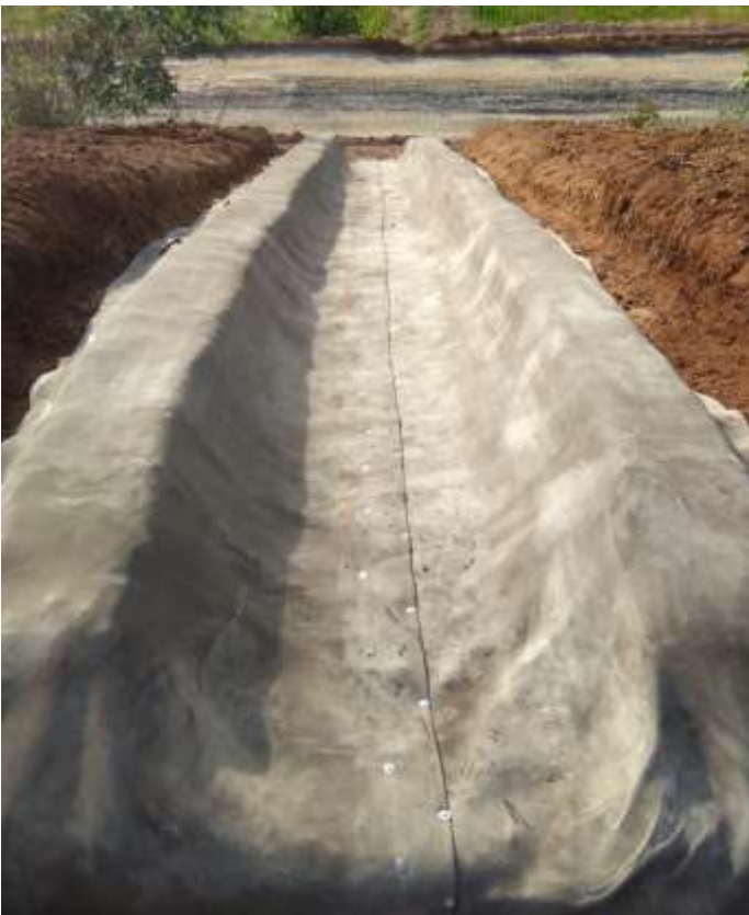
Fixing & Screwing Done
