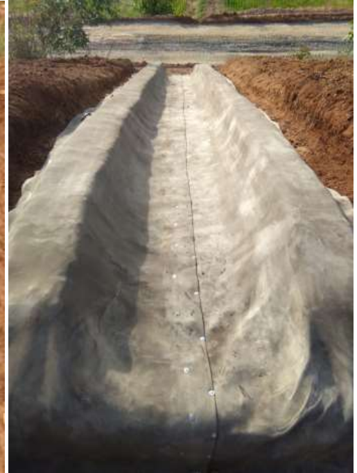
Installation Completion Photo
