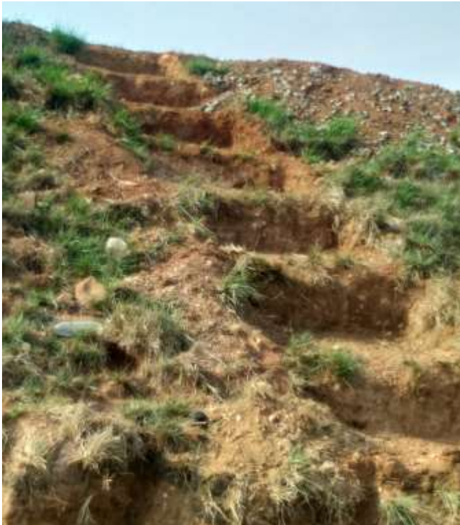
Before Photos During Site Visit
