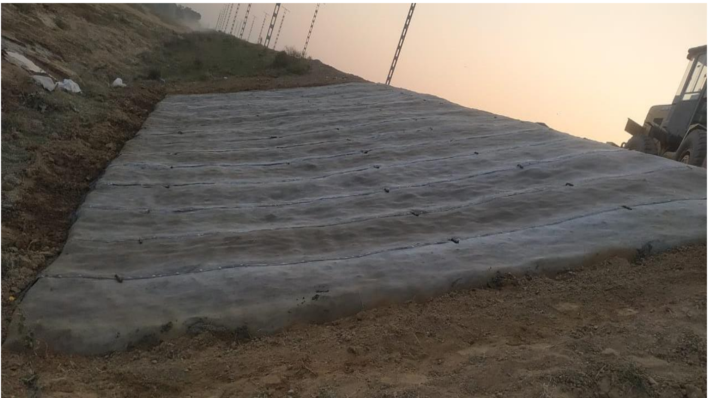
Installation Completion Photo
