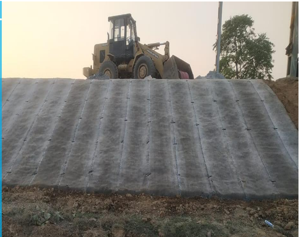
Installation Completion Photo
