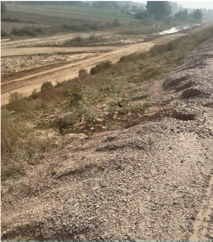
Eroded Slope & Rain-cuts
