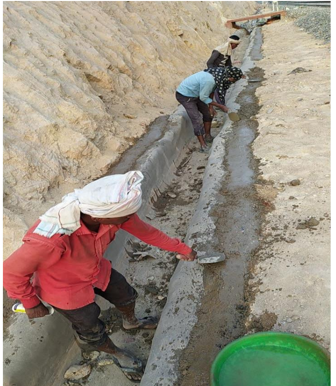
After Preparation done
