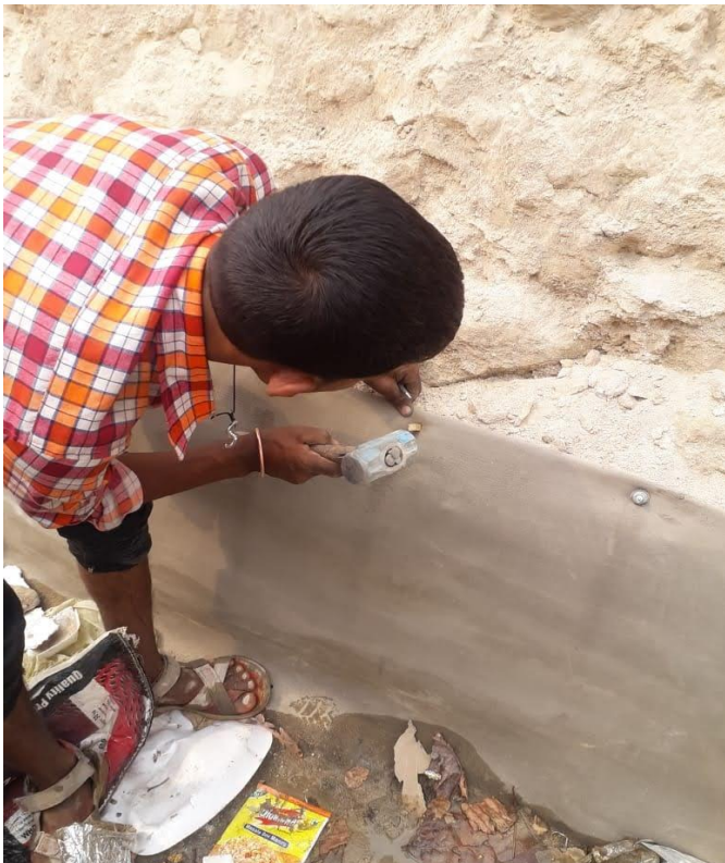
Sizing, Compaction & Collar work manually
