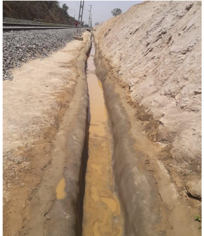
Laying of CC patches transversally
