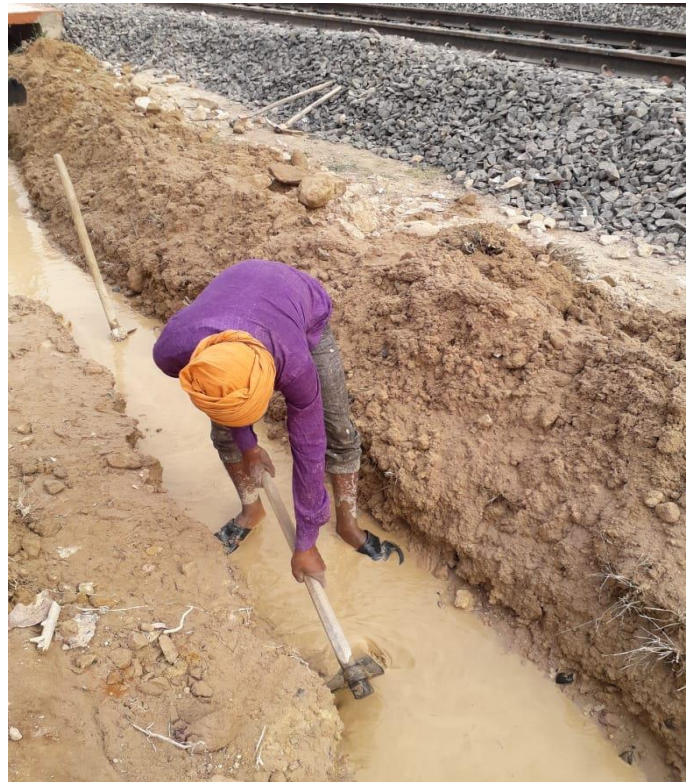
Excavation & Cleaning of Drain by JCB
