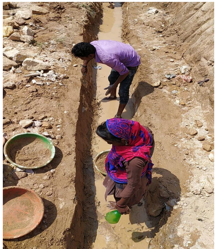
After Preparation done
