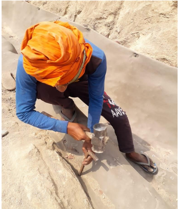
After Preparation done
