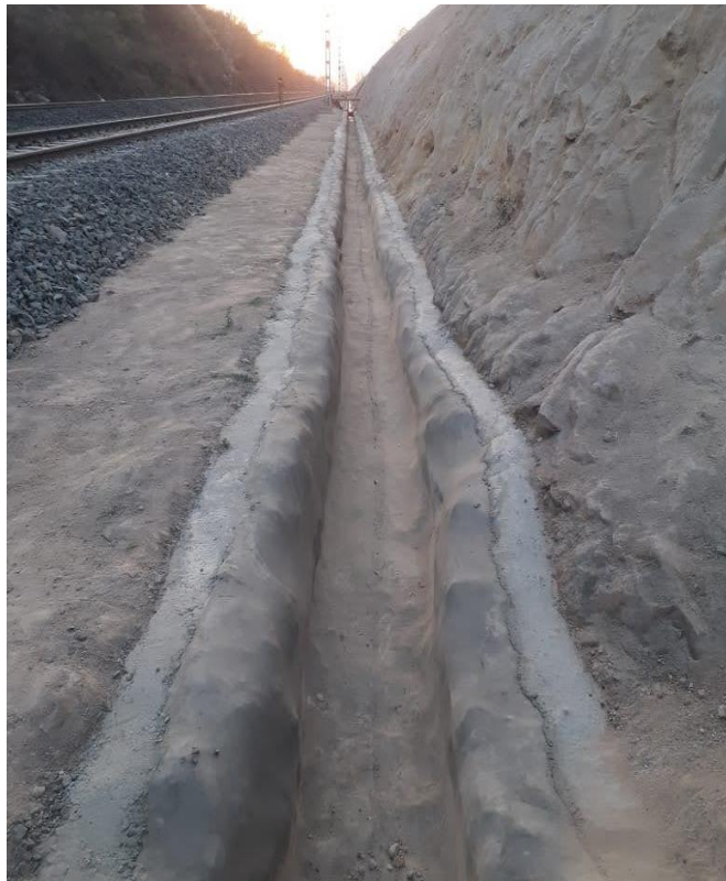
Screwing & Sealanting work Overlaps
