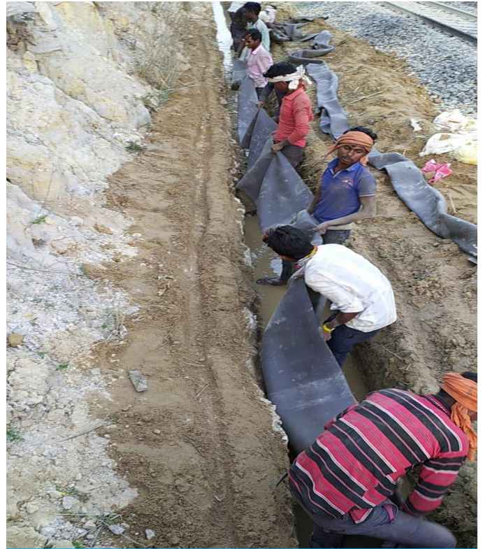
Excavation & Cleaning of Drain by JCB
