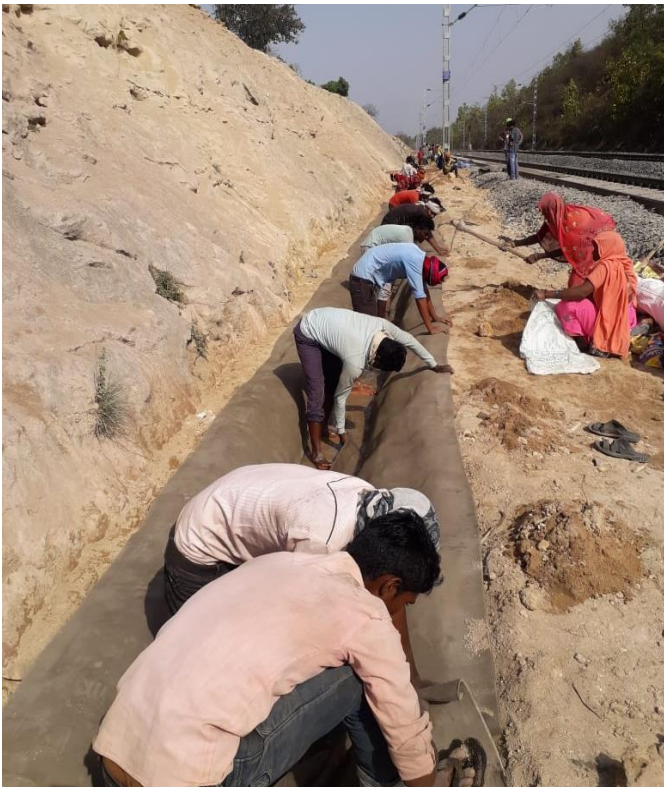
Sizing, Compaction & Collar work manually
