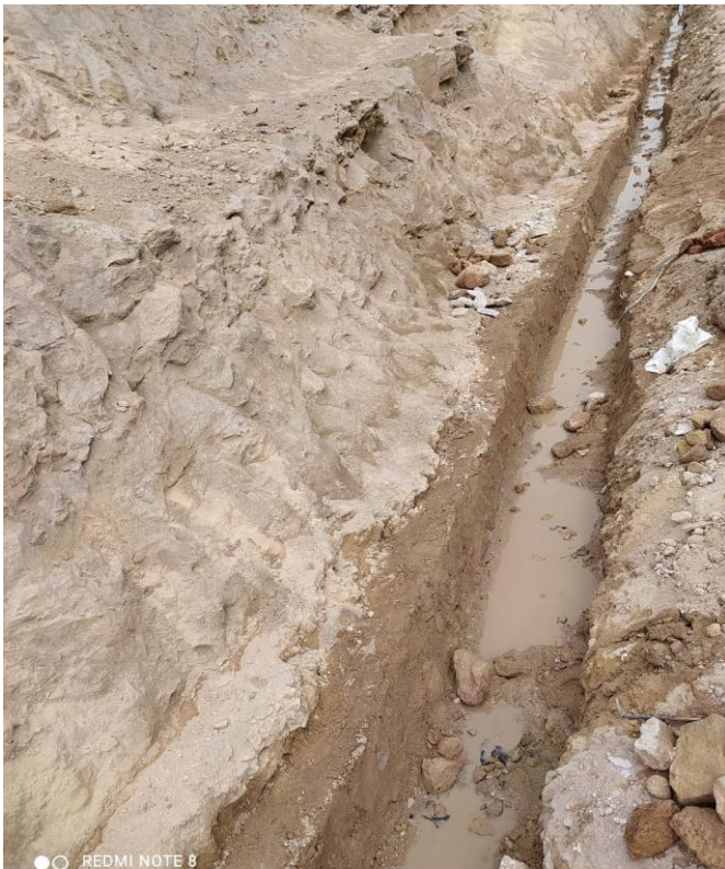
Sizing, Compaction & Collar work manually
