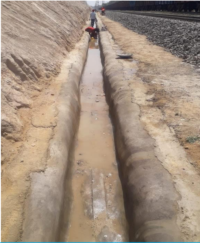
Starting Edge of Drain
