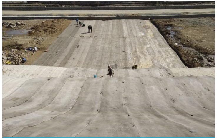
Complete installation view from top of slope
