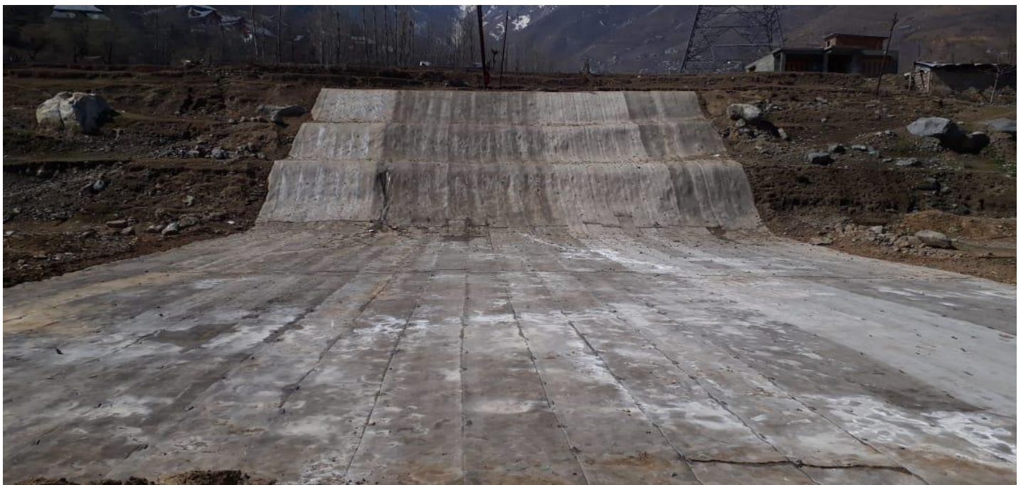
Complete installation view from top of slope
