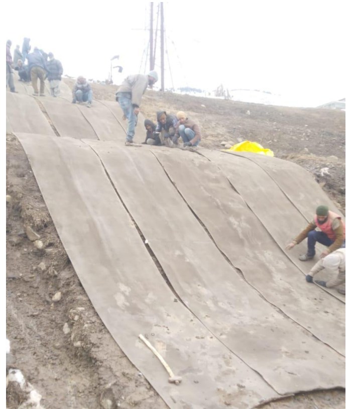
Laying of Concrete Canvas
