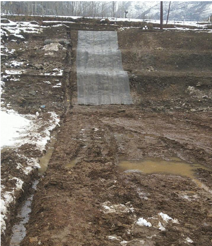
CC8 125sqm installation complete
