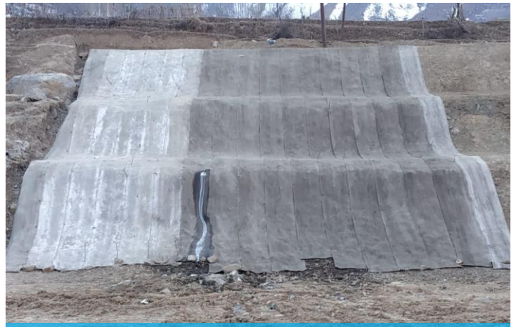
Complete installation on Slope area
