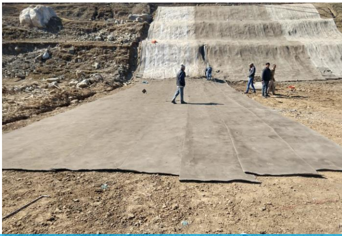
Laying on ground area
