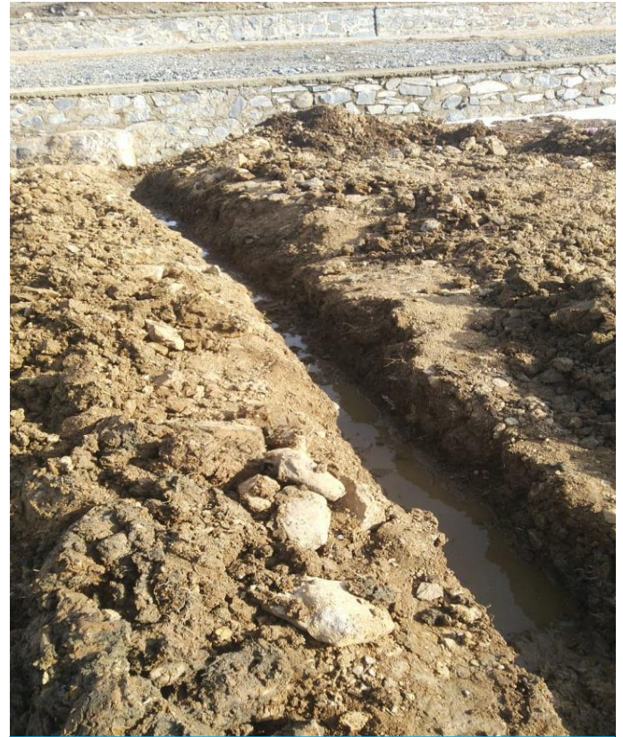
Side drain of slope
