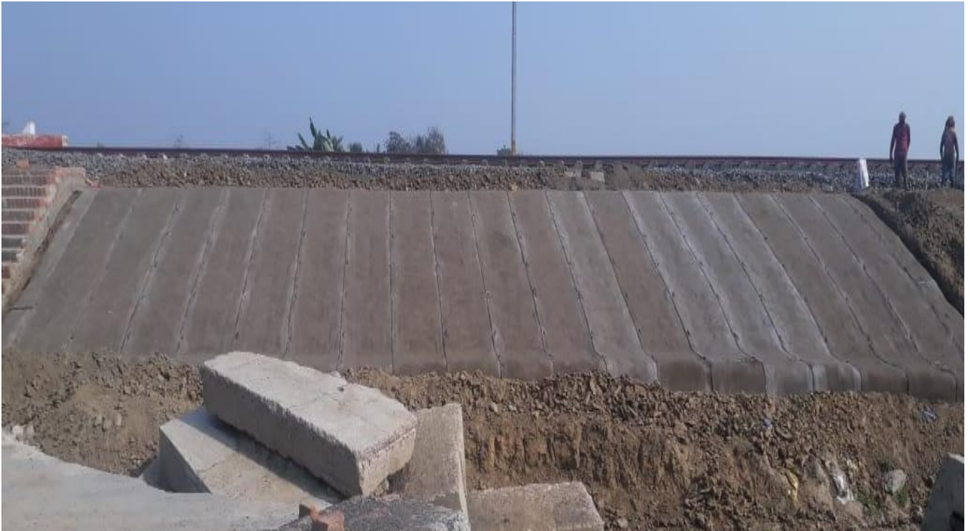
Location 2 Installation completed
