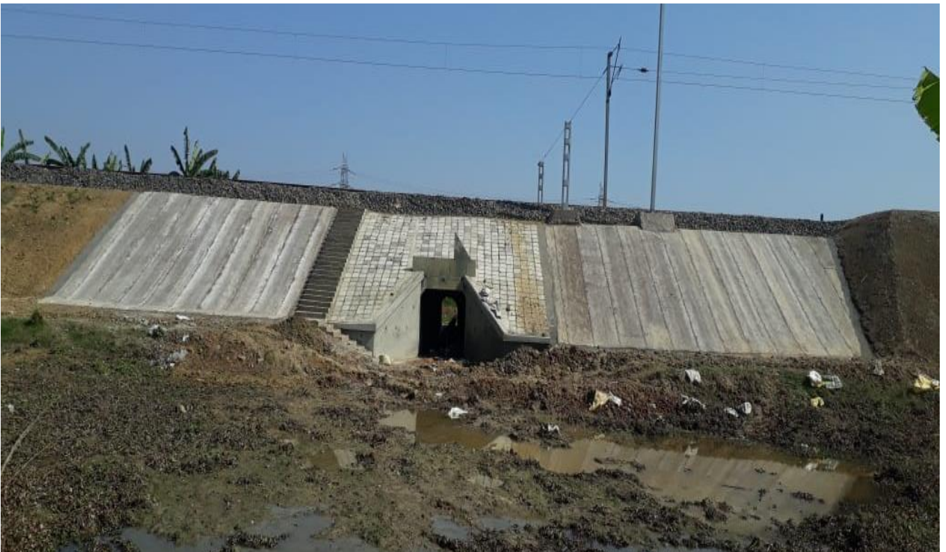
Location 3 Installation completed
