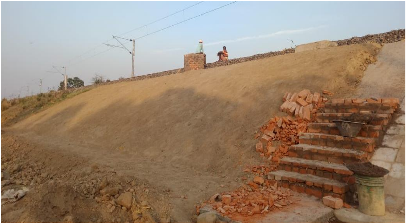
Laying of CC on levelled profile
