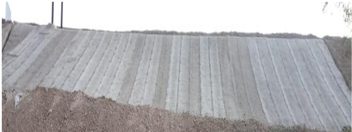
Installation Complete Photo
