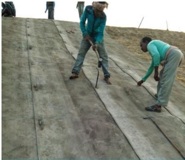
Pegging with spacing 1m
