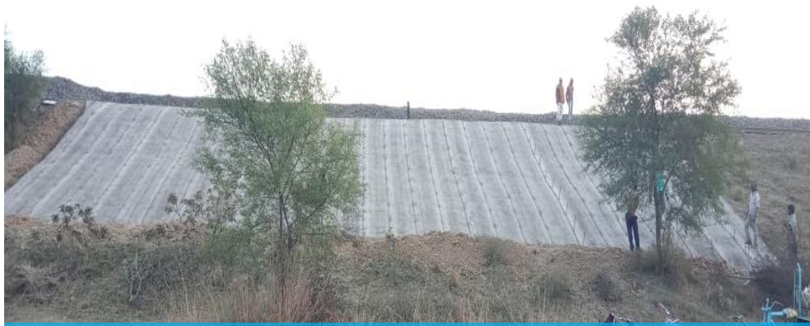
Installation Complete Photo
