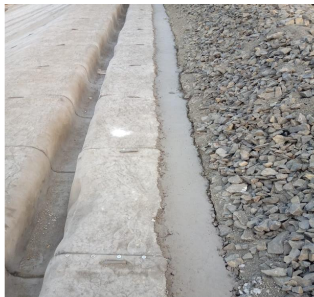
Concreting in anchor trench
