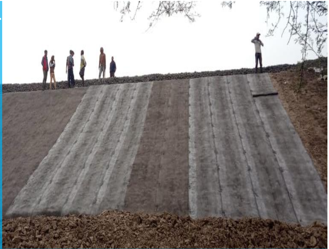
Working Installation Photos of Concrete
