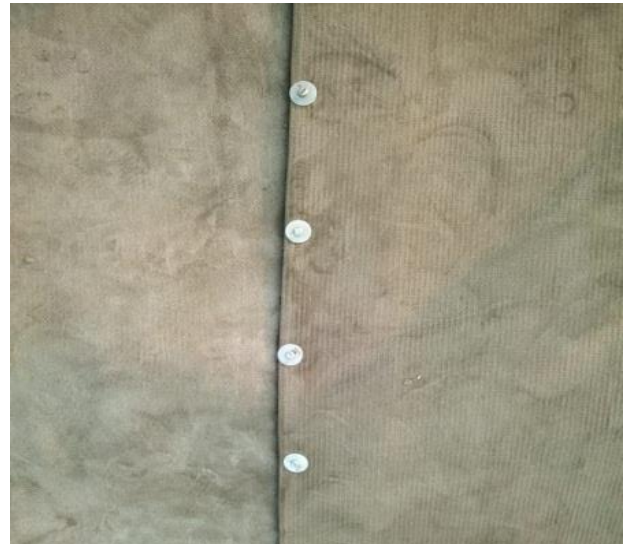
Screwing on 100mm spacing
