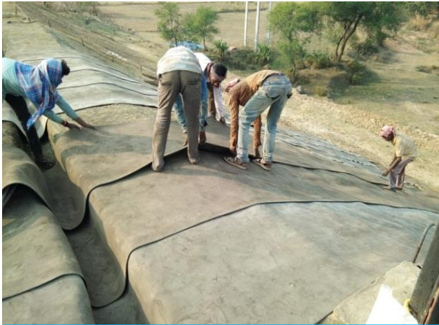
Laying of CC patches
