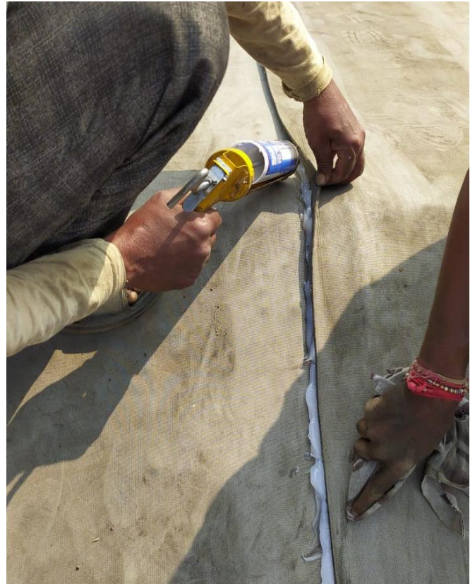
Edge sealing with silicon sealant
