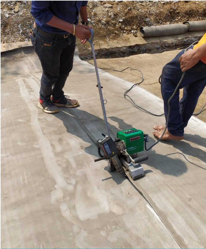
Jointing of overlap by thermal welding method
