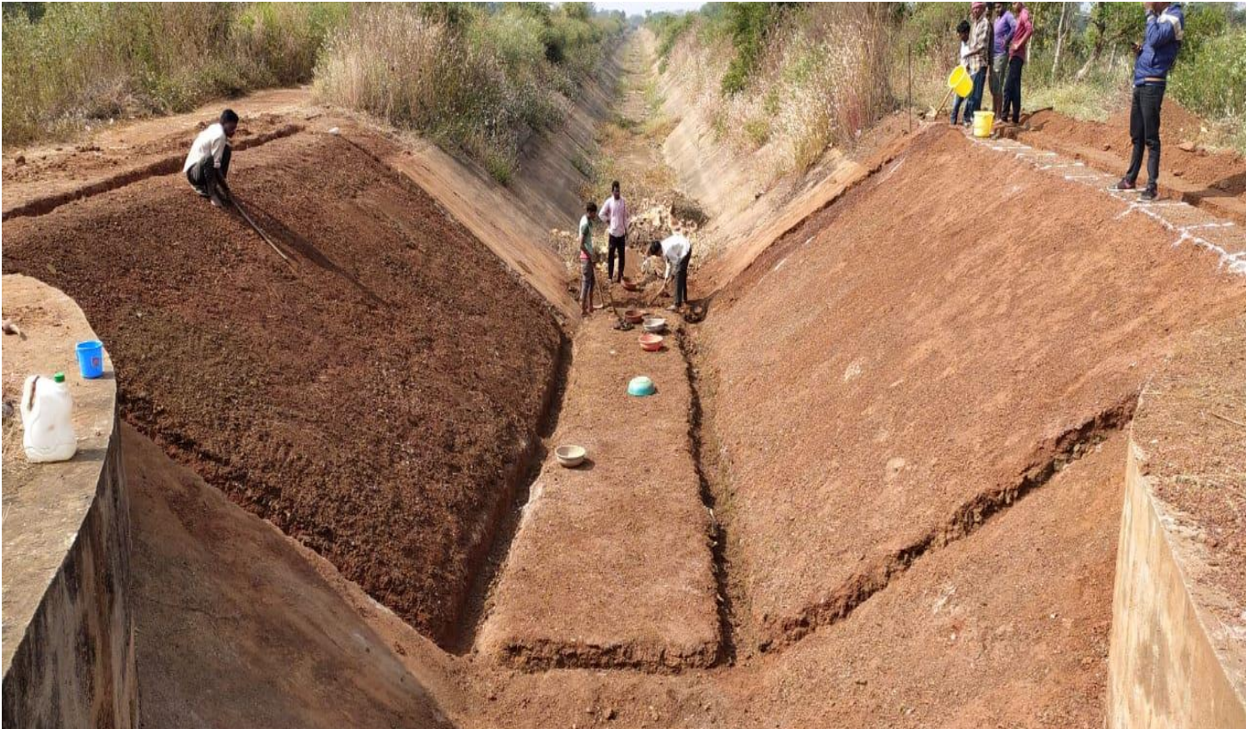
Preparation of canal
