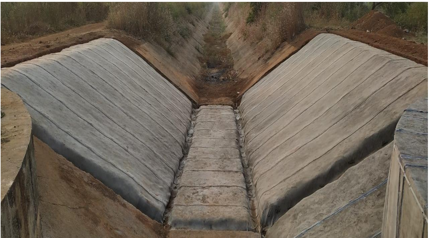
Completely lined canal with concrete canvas installation done at Location 1
