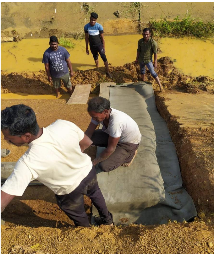
Laying of CC patches
