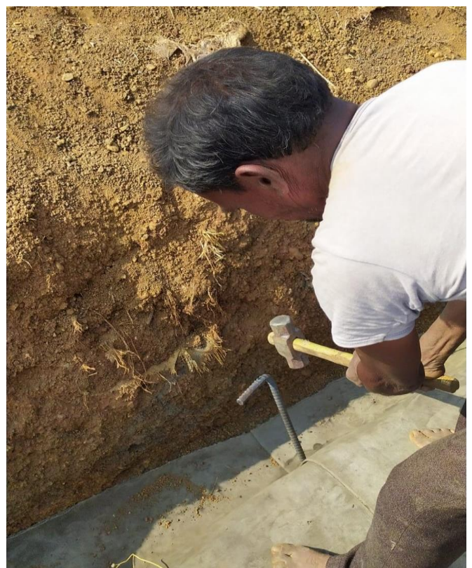
Fixing inside anchor trench
