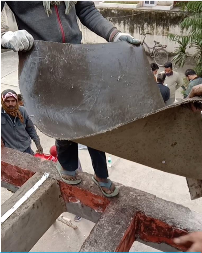
Placement of CC over beam
