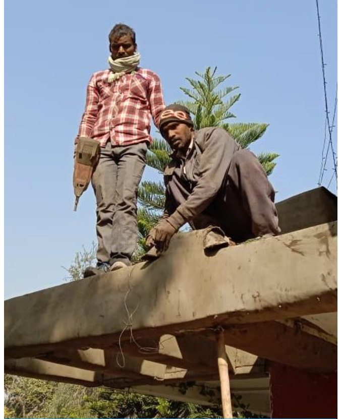
Hilti Nailing work
