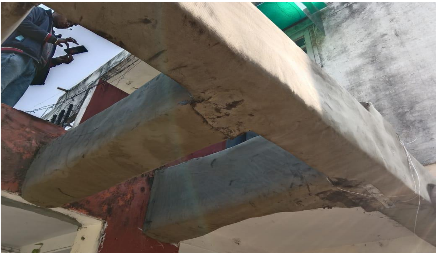
Bottom View of Completed Installation
