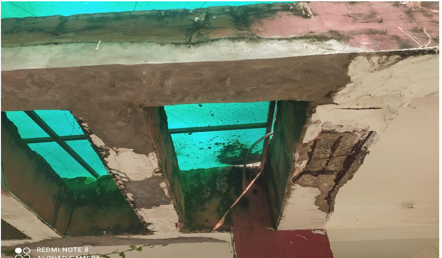
Initial eroded porch beams
