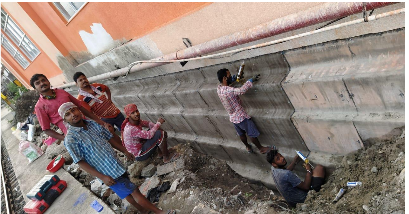
Labour team on Last day of installation.
