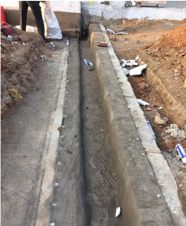
Complete installation with hilti & sealant
