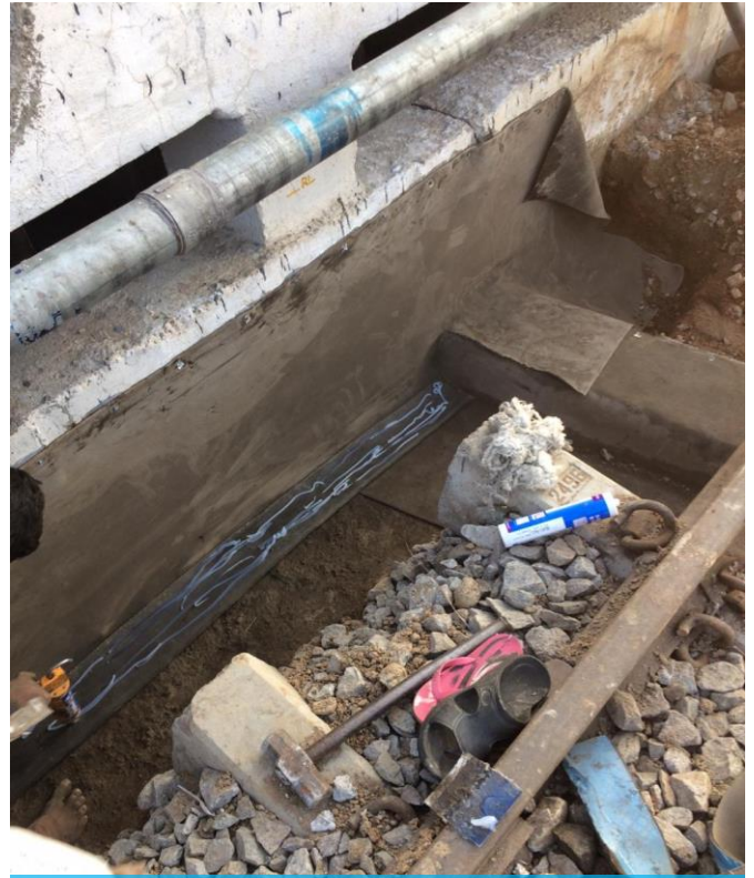
Sealant work on CC
