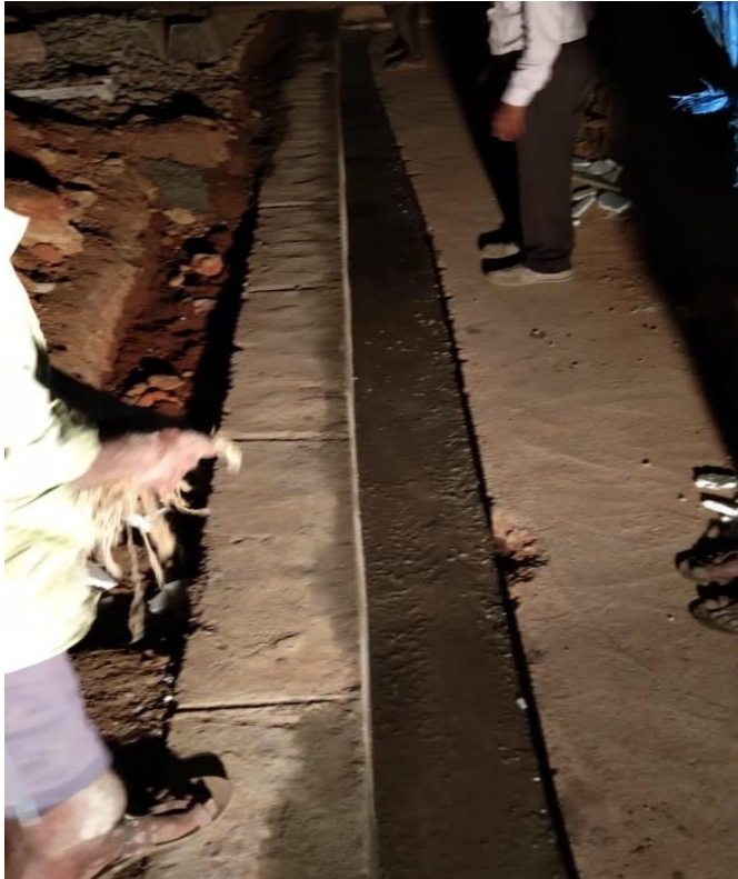
Filling of joints with concrete
