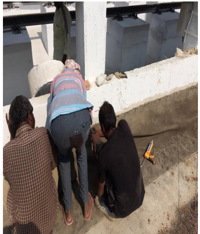
Fixing of CC with Hilti Nails
