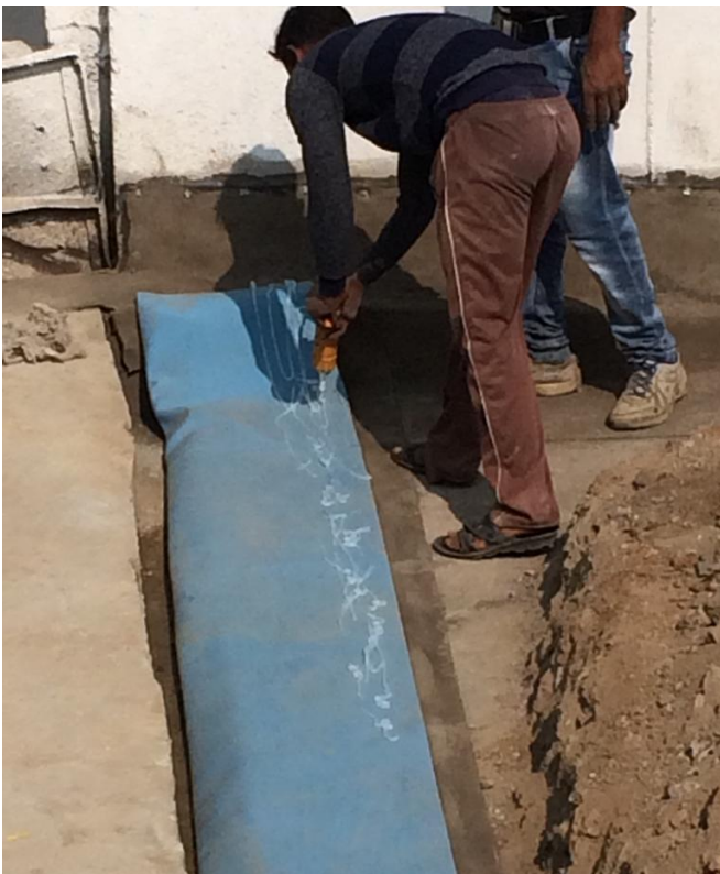
Sealant work on CCH
