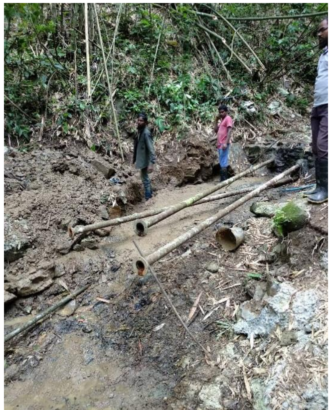
Fixing of piper inside soil to divert water on CC
