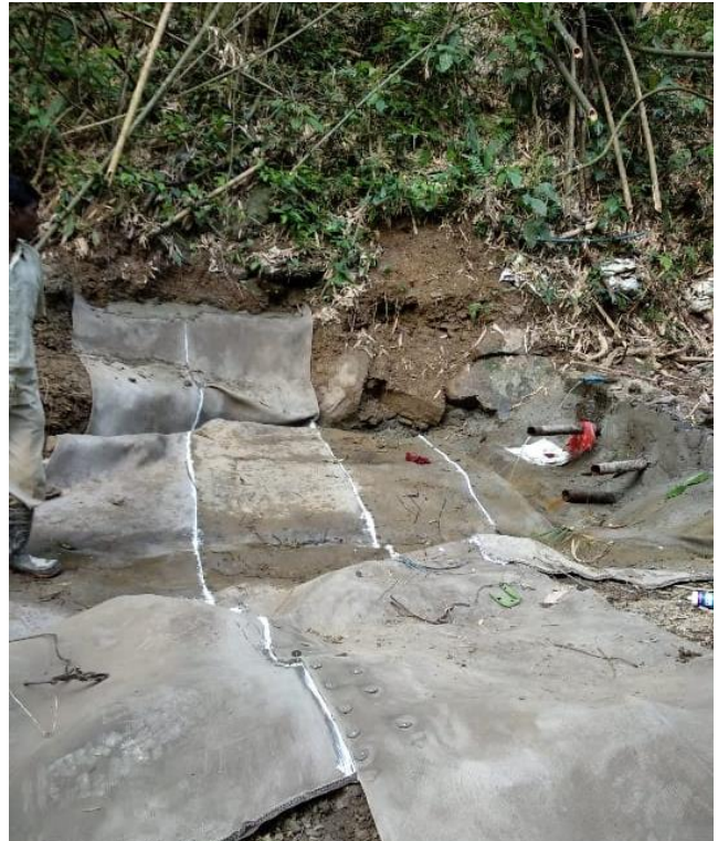
Laying and Joining of first 5m portion
