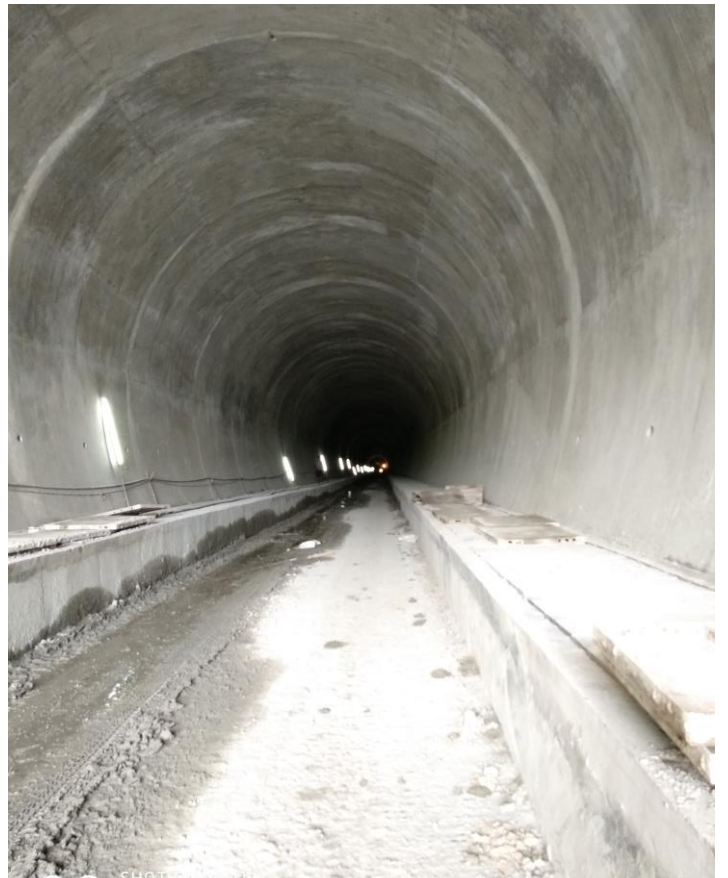
No leakages inside the tunnel
