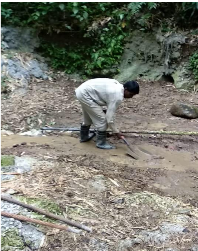
Cleaning of mud
