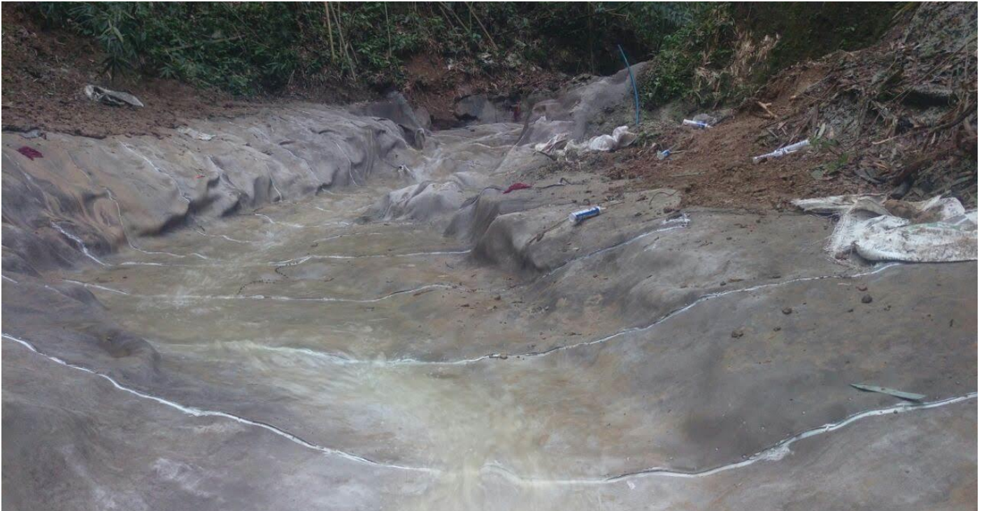
Completed installation after cleaning of site
