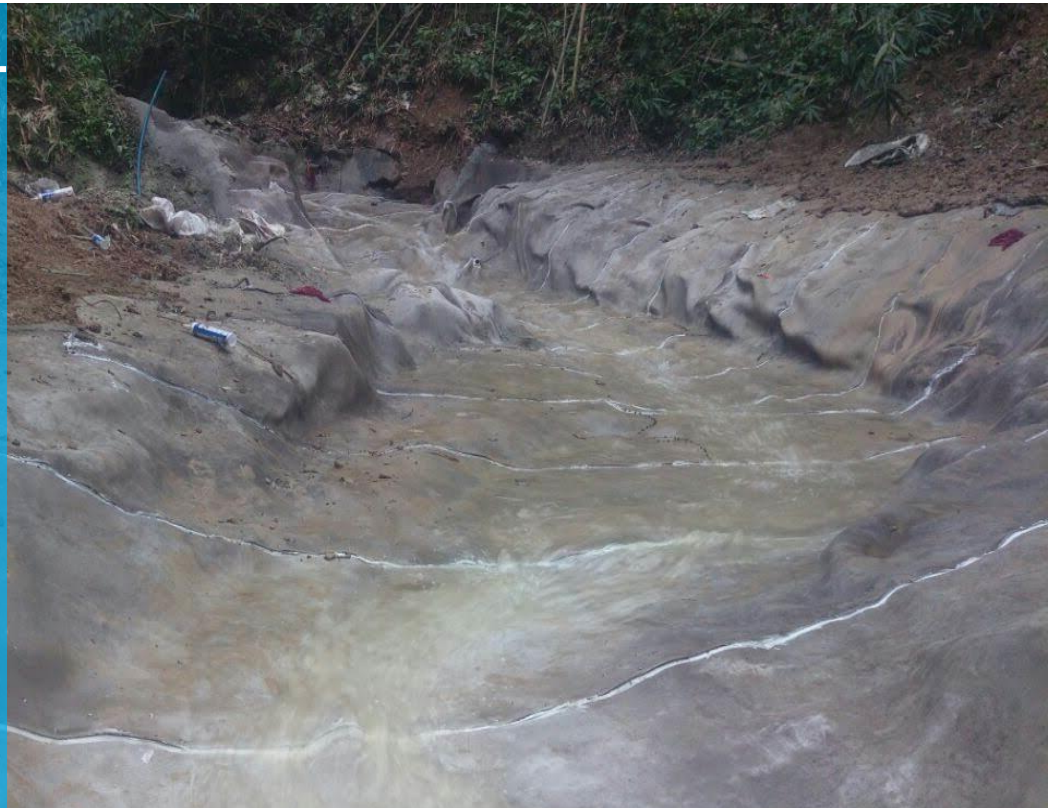
Channel formation to divert leakages from tunnel top
