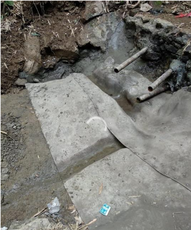
Laying of first patches
