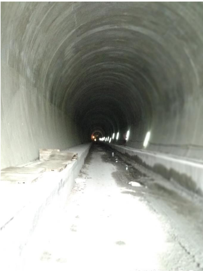
No leakages inside the tunnel
