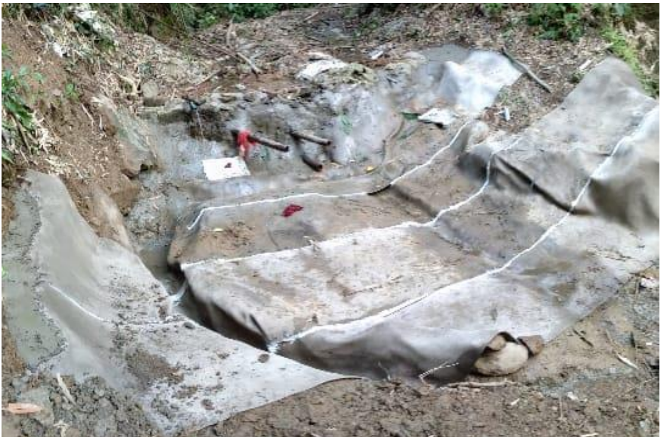
Front view: Laying and Joining of first 5m portion
