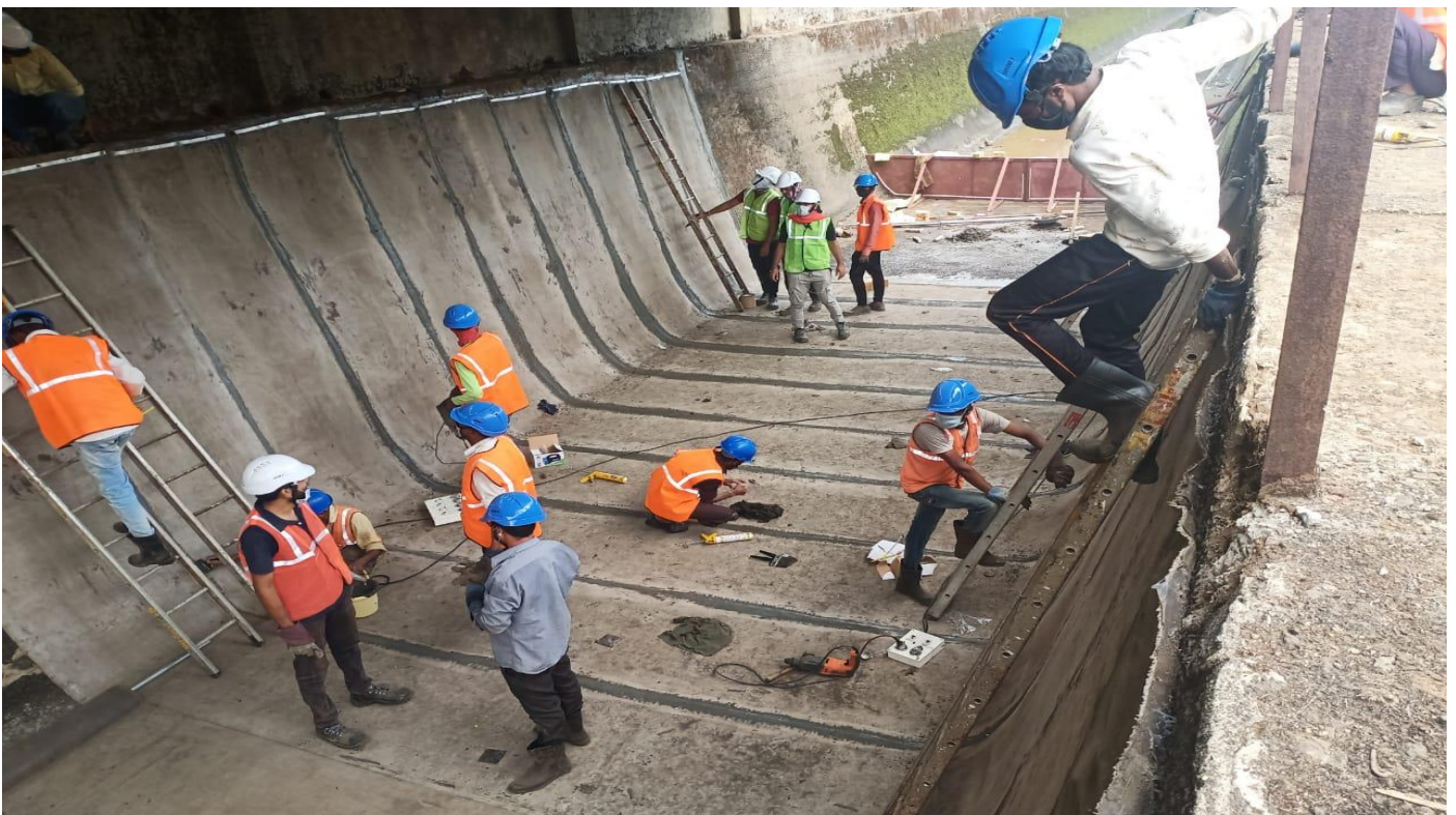
Installation of all patches
