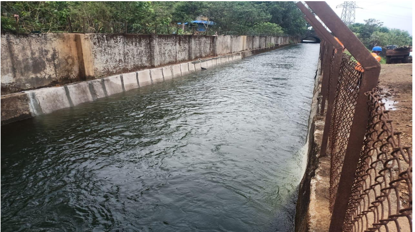
Full Supply Level after installation done in duct line
