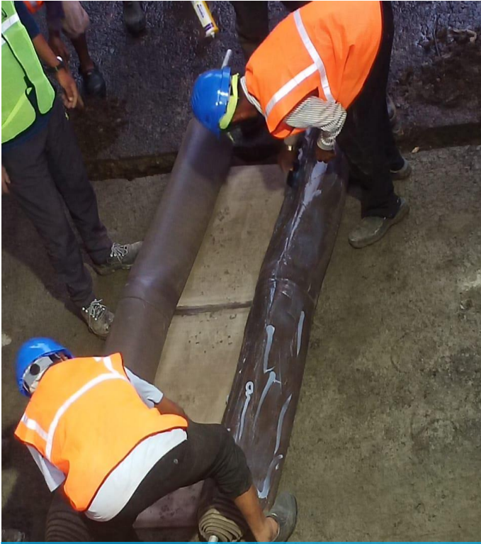
Unrolling from centre & sticking with surface
