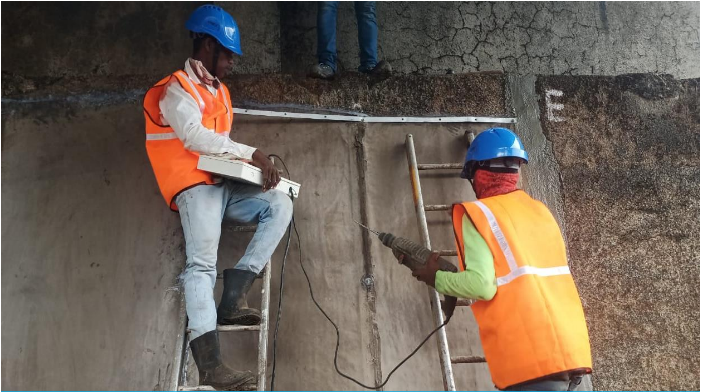
Anchor fastening on top edge
