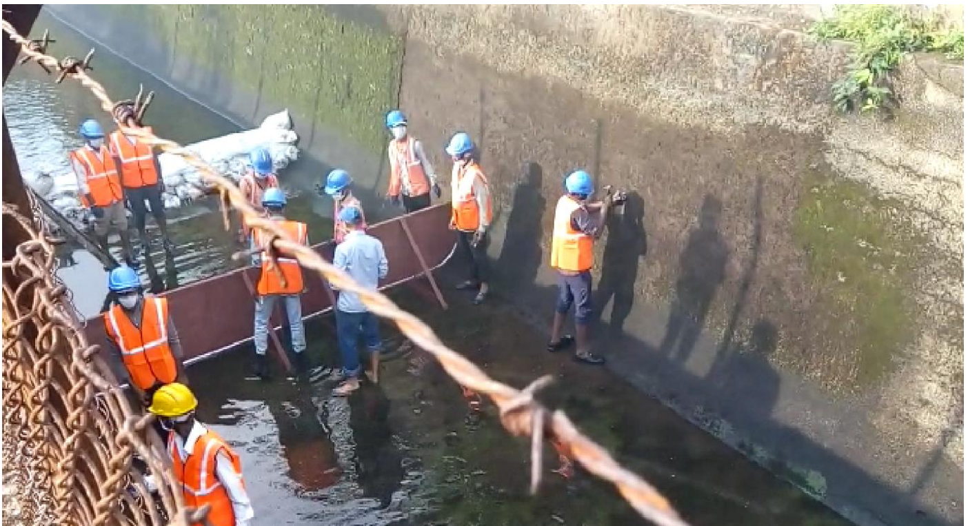
Dewatering of duct line
