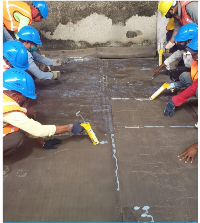
Sealant work on PVC portion
