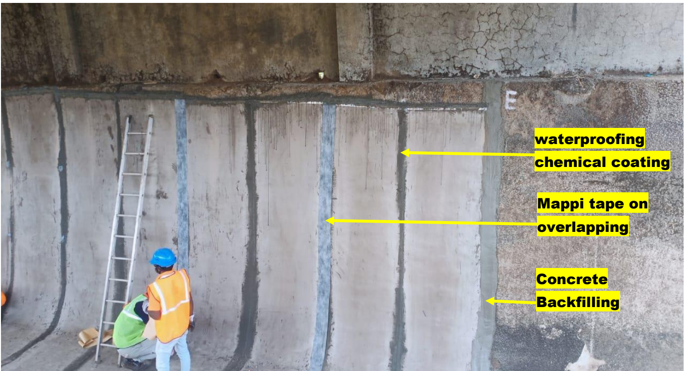
Overlapping securing with epoxy chemicals & stick tape
