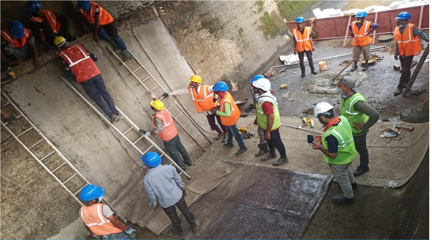
Similar installation of next patches
