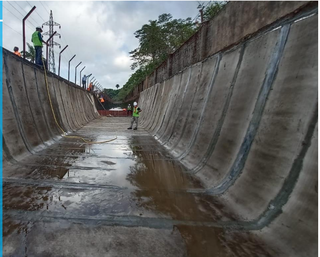
Work Completion photo
