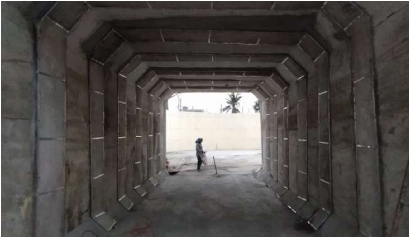
Installation Completed Site
