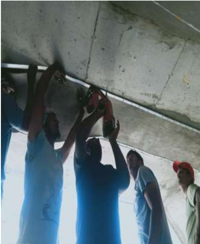
Fixing of top patch with Hilti nailing machine
