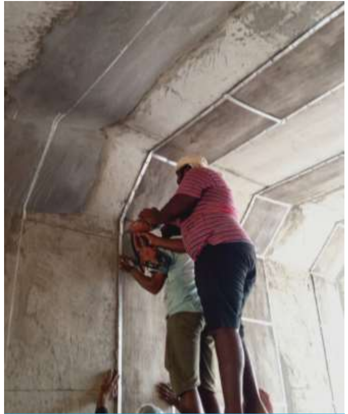
Fixing of vertical patch with Hilti nailing machine
