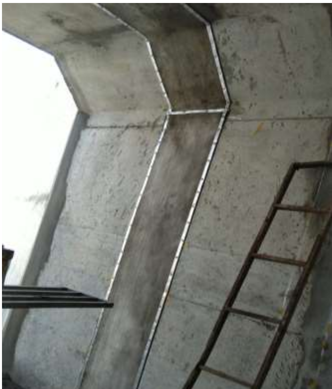
Fixing of vertical patch with Hilti nailing machine
