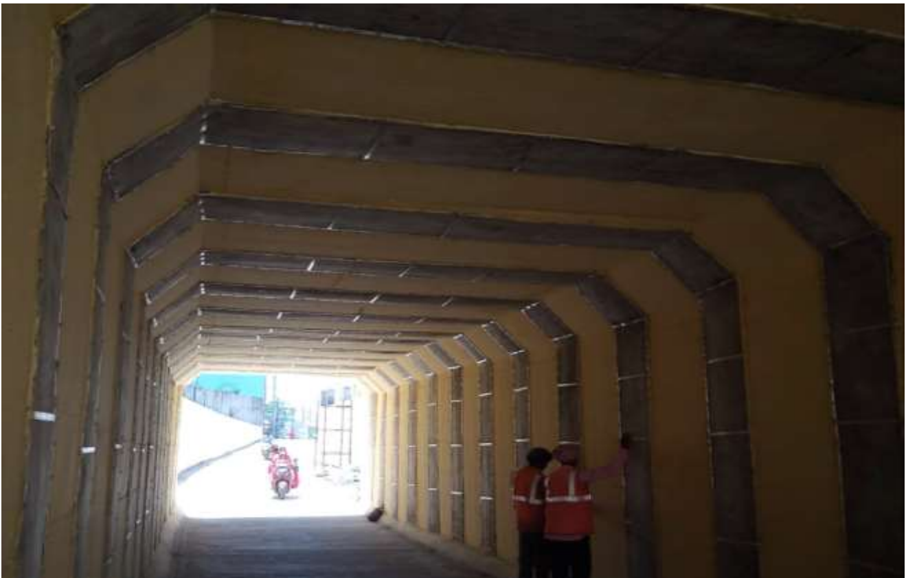
Installation Completed Site
